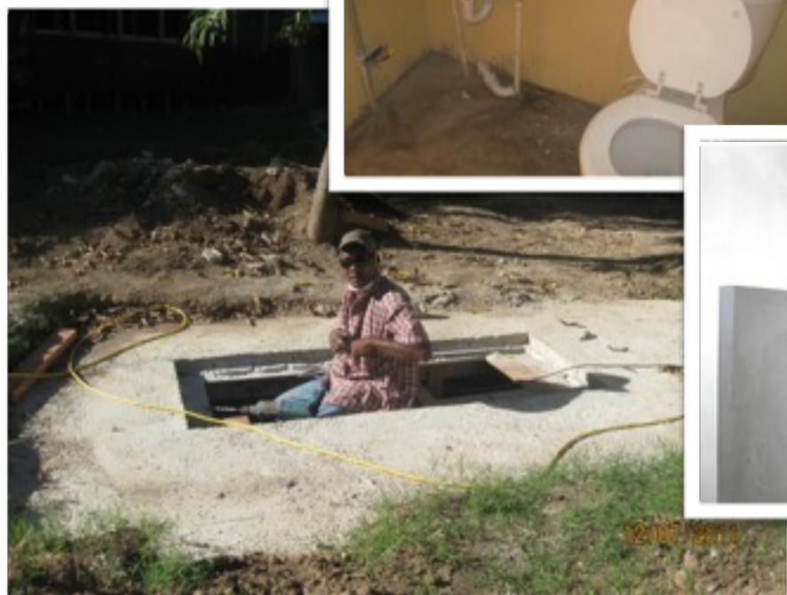
Septic field and tank for plumbing were installed to serve six bathrooms, 2 shower rooms, and sinks in each consultation room. Glass sliding windows, fans and lights are installed.
