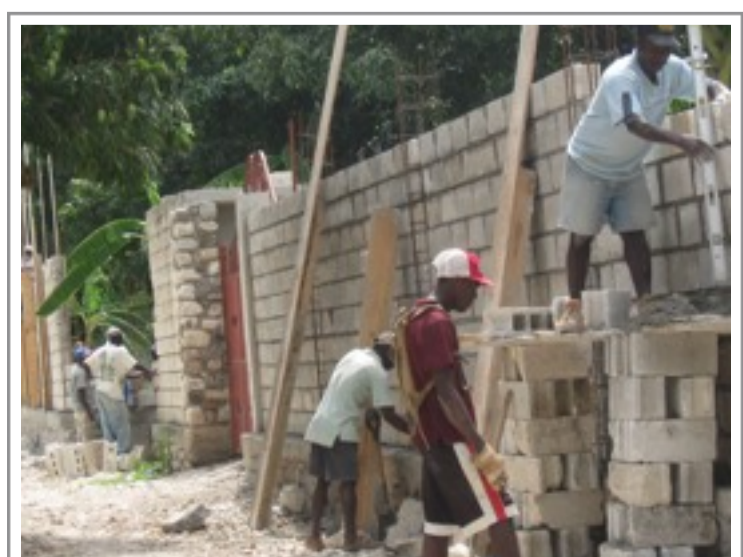
↑The construction of the temporary elementary school building, included 7 classrooms and an office, was aided by the new skid-steer. ↑ ↓The new wall was reinforced with rebar ever six inches in the block and surrounded the whole 5 acre property.
