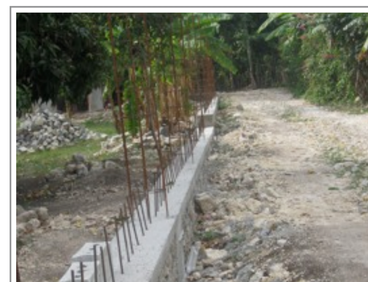
↑The construction of the temporary elementary school building, included 7 classrooms and an office, was aided by the new skid-steer. ↑ ↓The new wall was reinforced with rebar ever six inches in the block and surrounded the whole 5 acre property.
